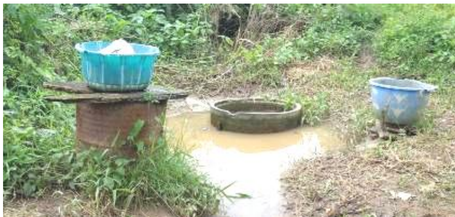
Plate 1: Hand-dug well (almost becoming a stagnant pond) as source of water in the Market area
