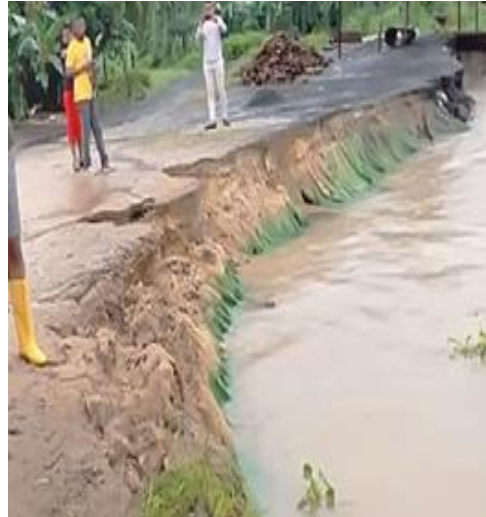
Fig. 4b. River shoreline erosion due to dredging near to shoreline at Obogoro community
