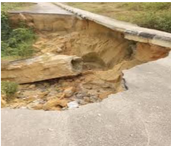
Fig. 3a. Road damage at Tombia caused by heavy vehicles laden with tonnes of sand
