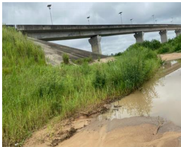
Fig. 3b. ground damage near Tombia – Agudama Ekpetiama bridge caused by heavy vehicles laden with tonnes of sand
