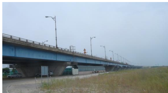
Figure 3: Side view of Sab-Kyo bridge
