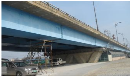
(b) Scaffold set-up and accelerometer installation
