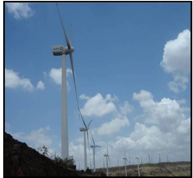
Figure 7: Wind farm located in hilly region
