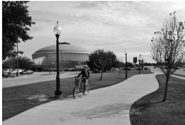
Figure 4: View of Completed Pedestrian and Bike Path with Acorn-Style Pole Fixtures and Pavement Surface LRV of 39%
