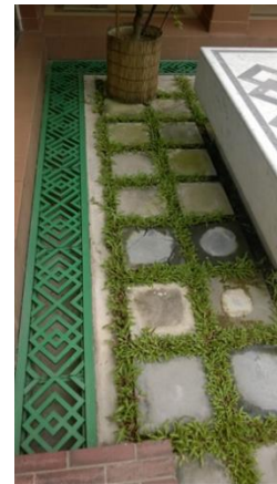
Figure 6: Peripheral gutter in the roof garden of Jamatkhana, Bashundhora R/A using design detail type 2 green roof
