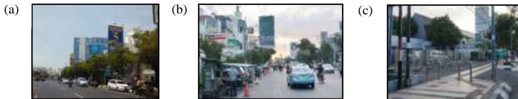
Figure 2. (a) Trees as a shelter; (b) The parking system at the street; (c) The condition of the pavement
