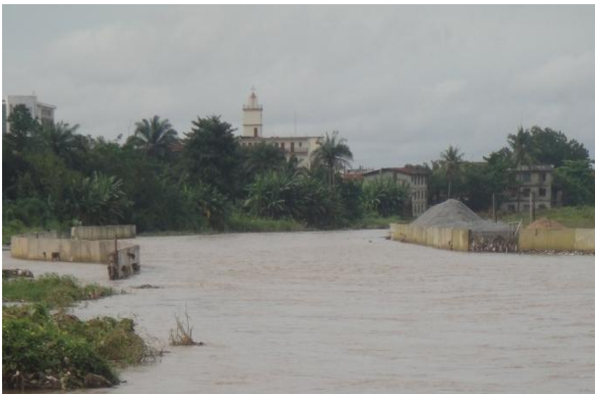
Figure 5: Construction of flood prevention structure along Asa River at Maraba.
