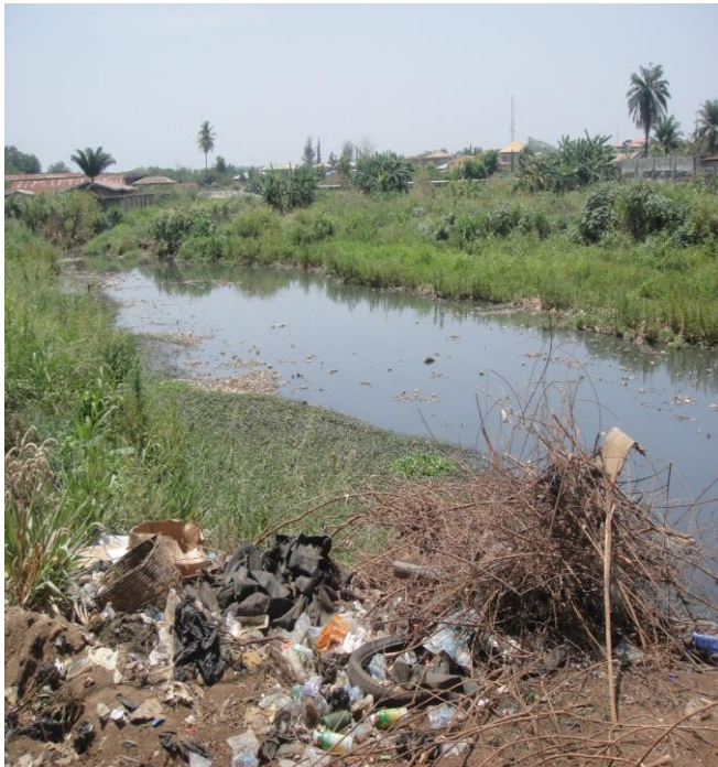
Figure 4a: Vegetation growth in the river channel of Asa River at Unity road, Ilorin (before rainfall).
