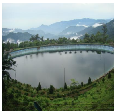
Fig.5 : Water harvesting through interrelated channel pipe rain water (Alagariah, 1600 m asl)
